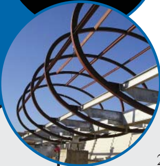
Field photo of the walkway portion of the Dos Lagos Project.
